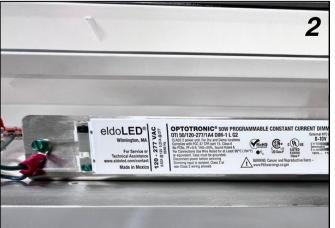
2. Before wiring the new driver, inspect driver diagram (H) and wire accordingly.
