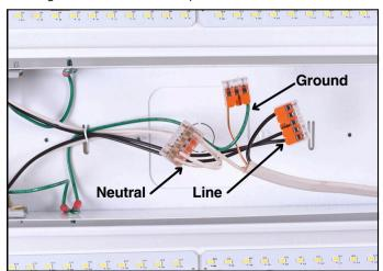
7. For surface installation, carefully tuck wires into housing, install cover (G) and screws (F).
