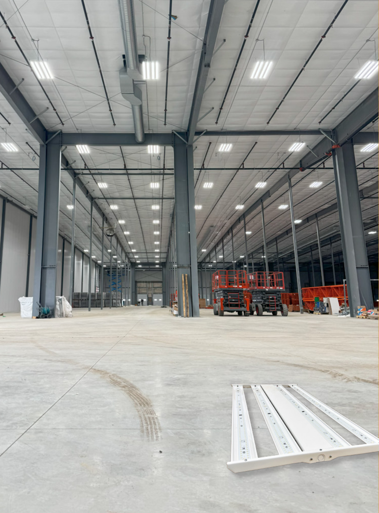
BAS-2X4 Linear Highbay 5000K | Suspension Mounted Motion Sensors
